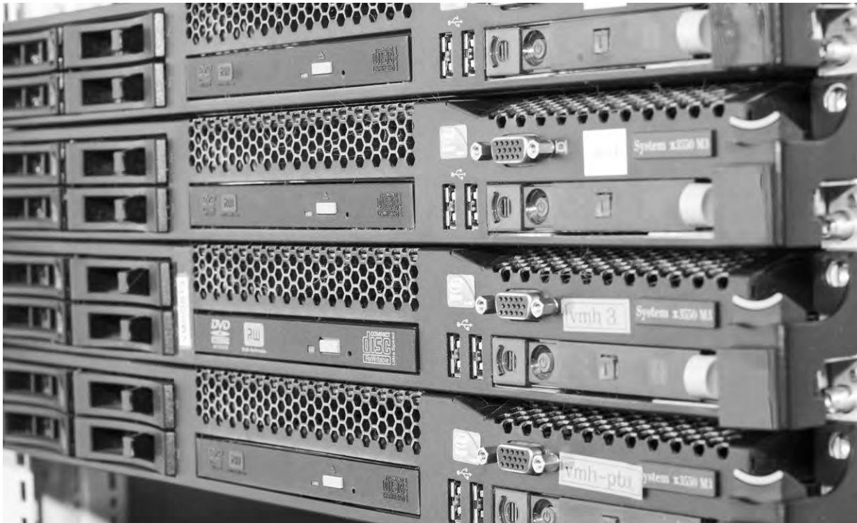
... to digital mass storage racks
